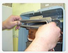
3. Remove the inside three screws from the flue terminal and set aside.
